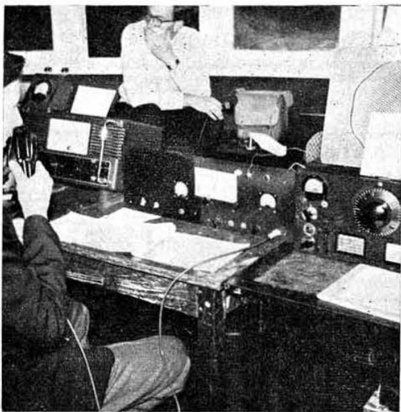
The Reigate Amateur Transmitting Society operated G3MHD/A on 144 Mc/s, G3NKS/A on Top Band and G3JDN/A on 7 Mc/s at the Reigate Grammar School Summer Fair. Equipment included an SCS22 and Vanguard transmitters and HRO, R208 and S640 receivers. The aerials were a 4-over-4 and 150 ft. end-fed wire.
